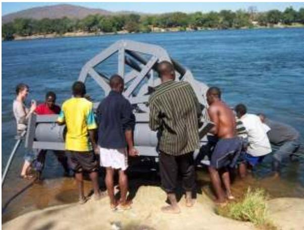
**Deploying the Waterwheel Pump on the Zambezi River**
