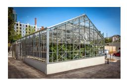
The Emory University WaterHub isn't a typical treatment facility. It filters wastewater through plant roots and microbes clean out organic material...A model for us all!
