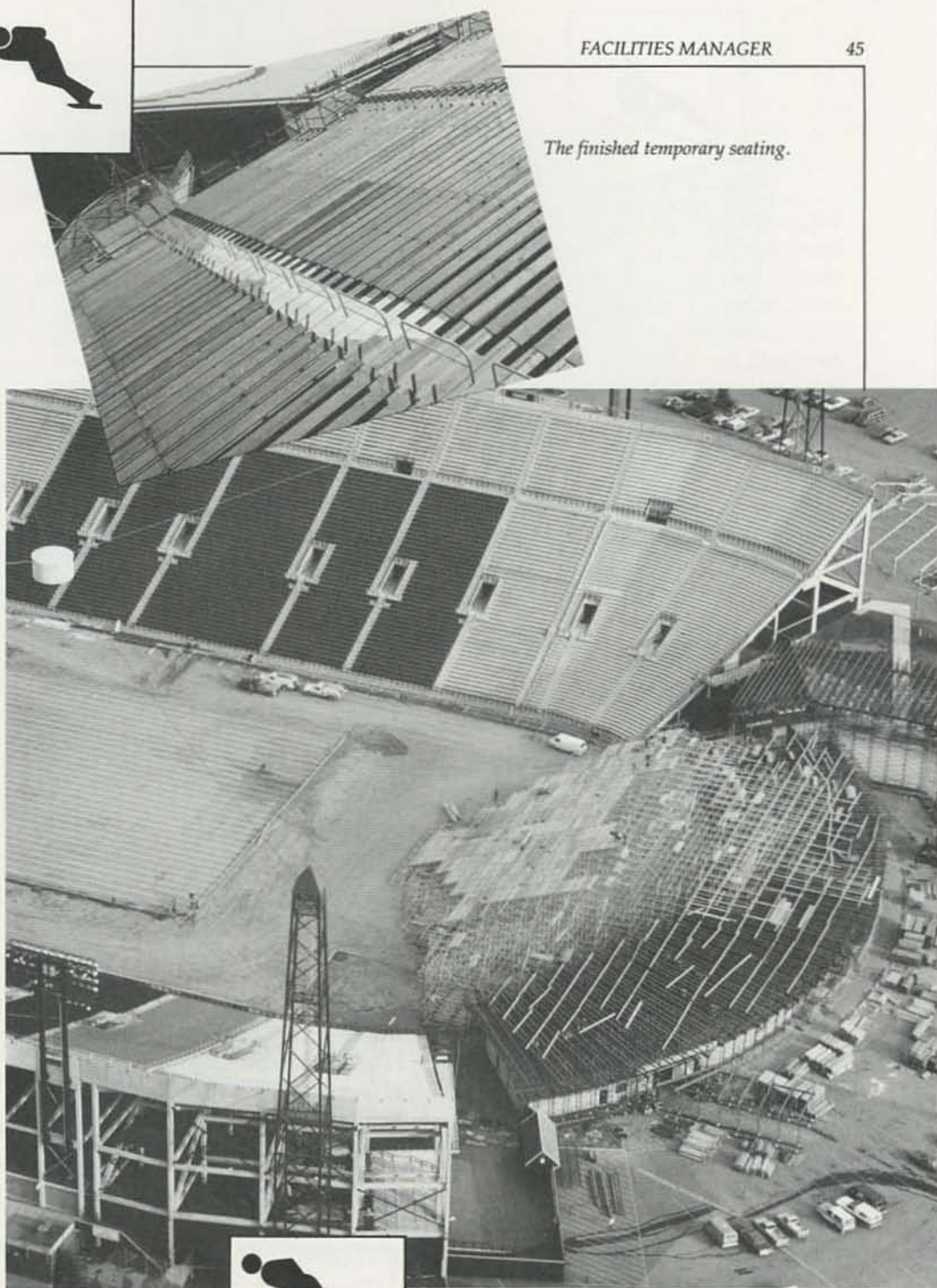
Temporary seating showing the special trusses used to span the buildings and to build tunnels to provide access for parading athletes and floats.
