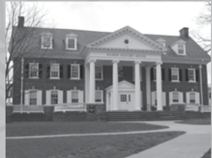
Lafayette College Interior Adaptive Reuse
