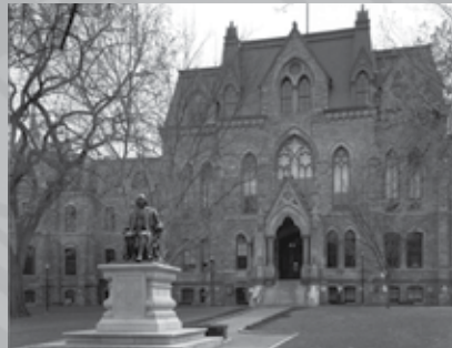
University of Pennsylvania Historic Stone Facade Repairs
