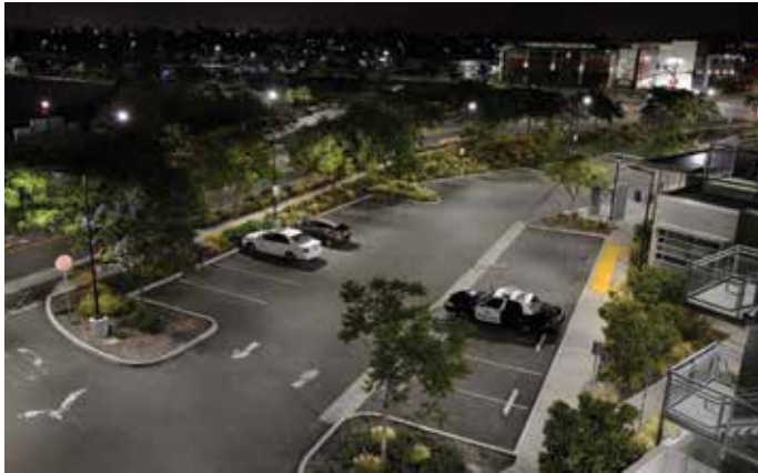
LED lighting at SDCC.
