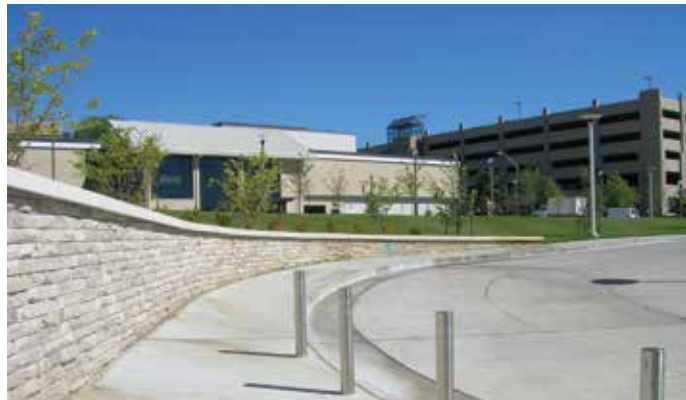
Salvages stone used in retaining walls at Pershing Commons.
