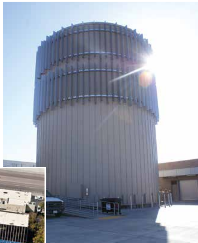
Above: Thermal Energy Storage Tank at San Diego Miramar College.
