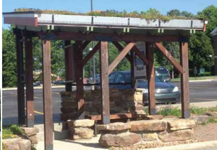
A joint project by students and the facilities planning department, the Green Bus Shelter is made up primarily of recycled materials, and has a green roof.
