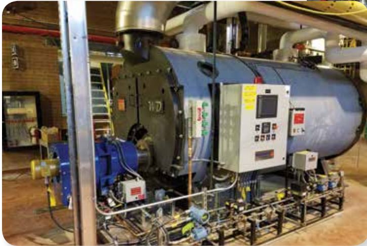
Left: Boiler side view with burner that can switch between "liquid wood" and natural gas. Above: All-stainless-steel boiler can process and burn "liquid wood."
