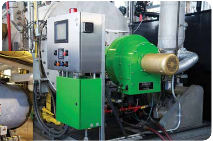
Left: Boiler side view with burner that can switch between "liquid wood" and natural gas. Above: All-stainless-steel boiler can process and burn "liquid wood."
