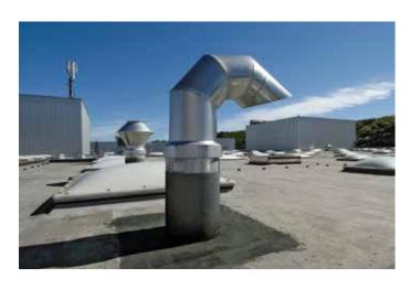
is an odor-free polyurethane (PUR) resin membrane system that is tinted throughout and color formulated to resist fading. Because there is no need to apply a separate topcoat over a membrane, the one-step application reduces labor and installation costs. To learn more, contact Kemper System at www. kempersystem.net.
