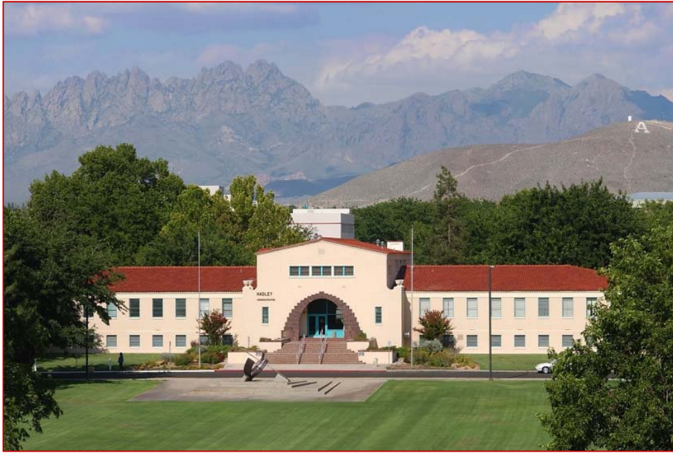
New Mexico State University Hadley Hall Administration Building
