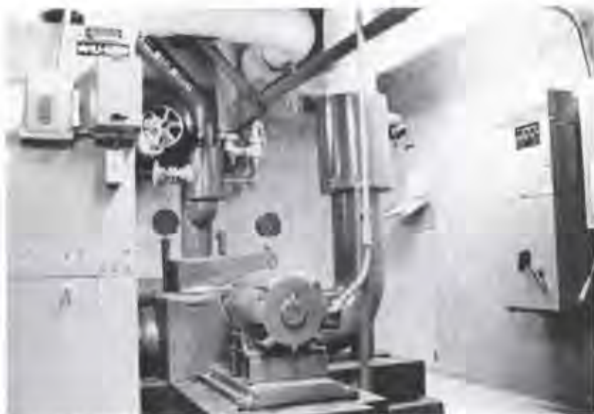
Building chilled water pump with Toshiba drive unit on wall.
