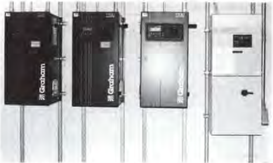
Variable speed drive with units for the cooling tower fans.
