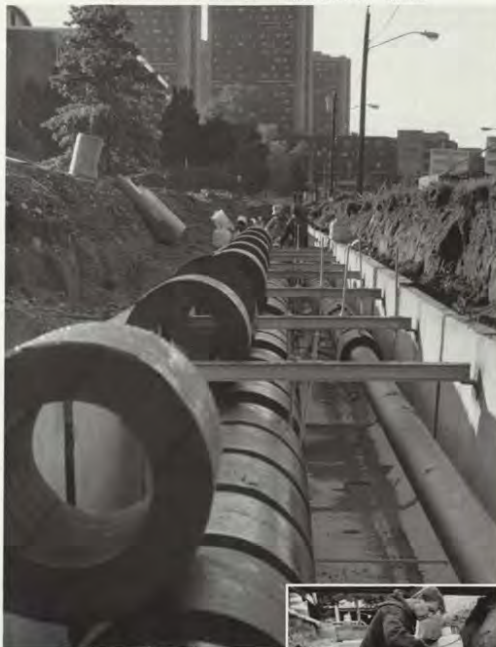
Live steam line (left) with StrataFab® insulation and jacketing; condensate return (right) prior to insulating. Inset: Prefabricated sections facilitated installation.
