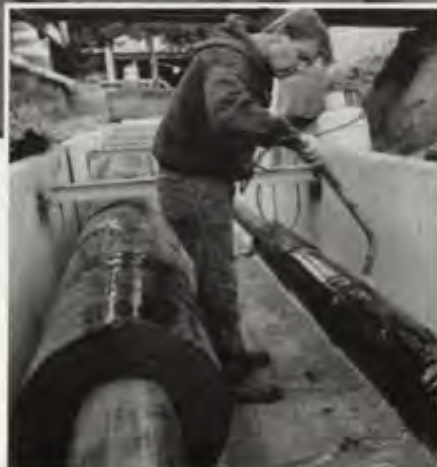
Live steam line (left) with StrataFab® insulation and jacketing; condensate return (right) prior to insulating. Inset: Prefabricated sections facilitated installation.
