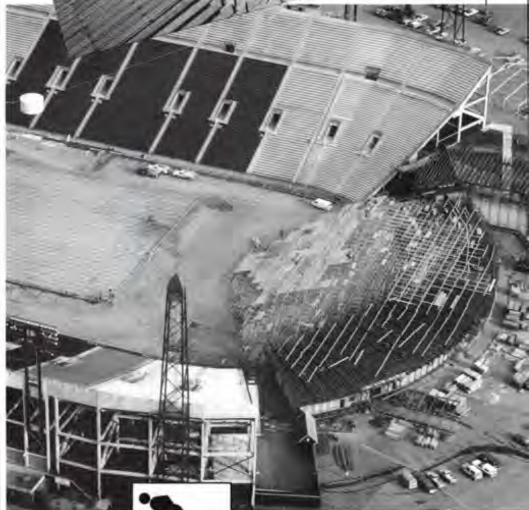
Temporary seating showing the special trusses used to span the buildings and to build tunnels to provide access for parading athletes and floats.
