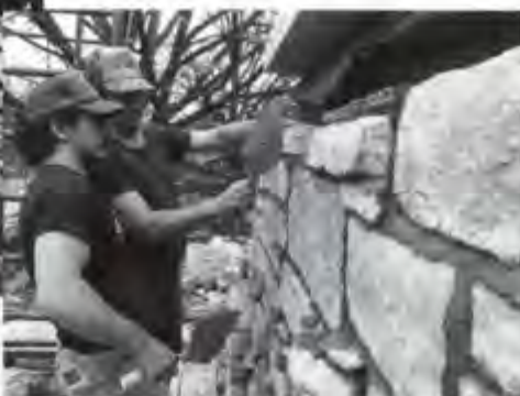
Stone masons are moved around several times daily to avoid unconscious patterning.
