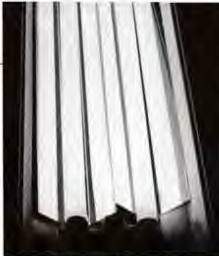
Close-up of fixtures in 306 Lewis Hall with silver reflector. Note the two lamps and four reflected lamp images.
