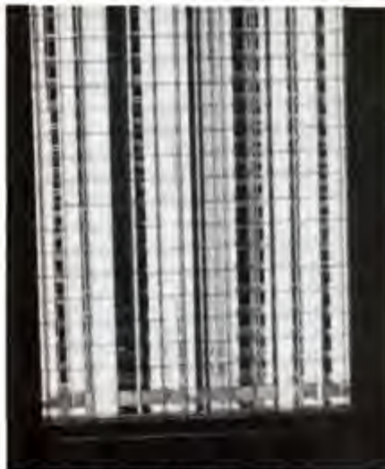
Close-up of Sproul Hall fixture with silver reflector and parabolic louvre.
