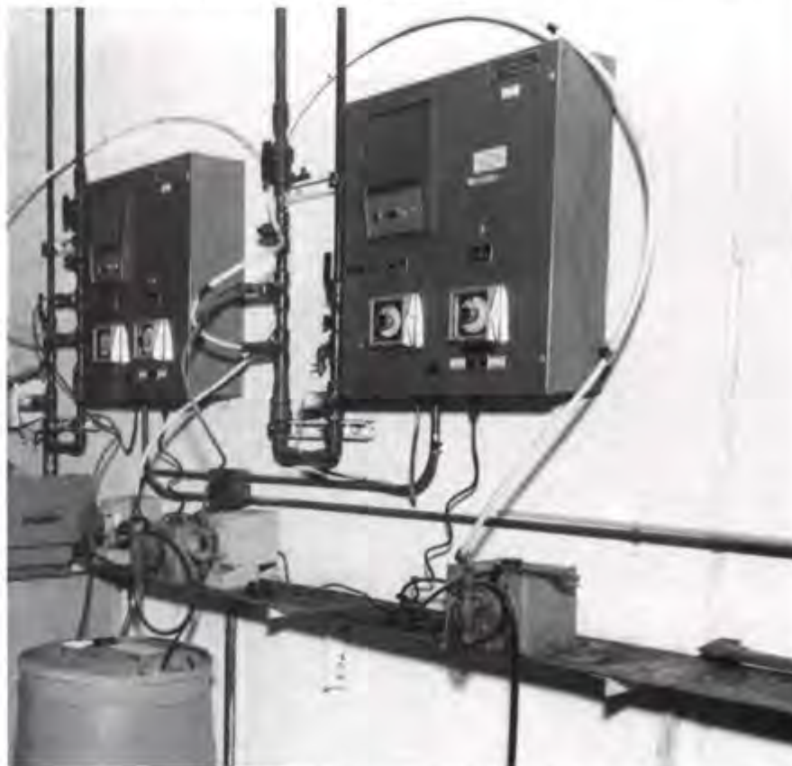
Monitor units serve the "open" cooling towers of the chiller plant.
