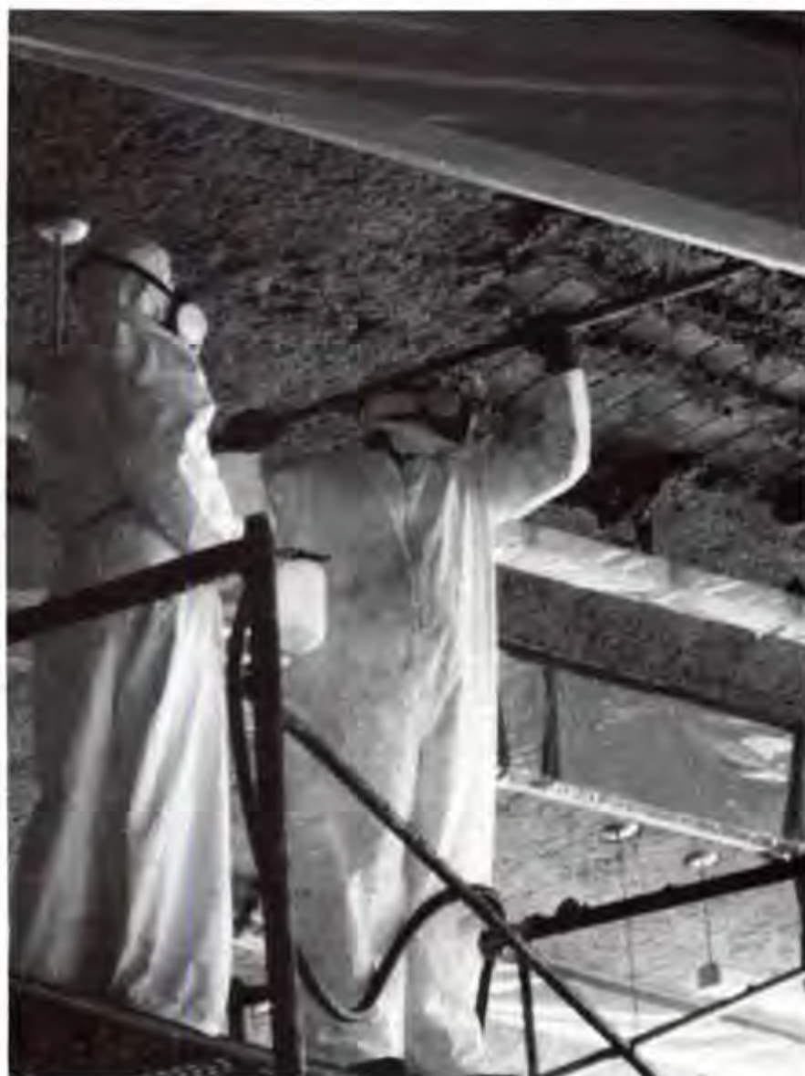
Workers removing asbestos from ceiling.
