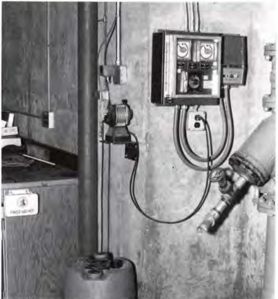
Conductivity monitor for "open" cooling tower. Monitor is located in basement mechanical room of three-story communications building.
