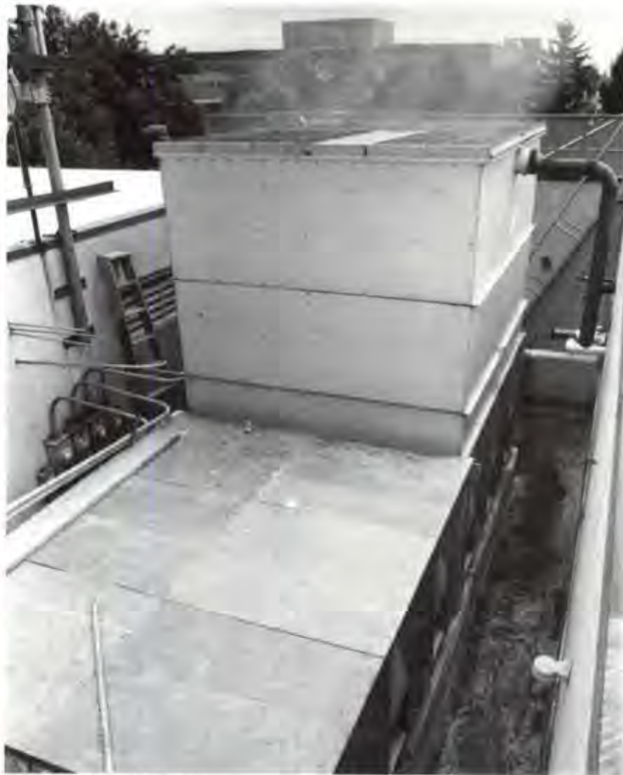
One of two "open" cooling towers.
