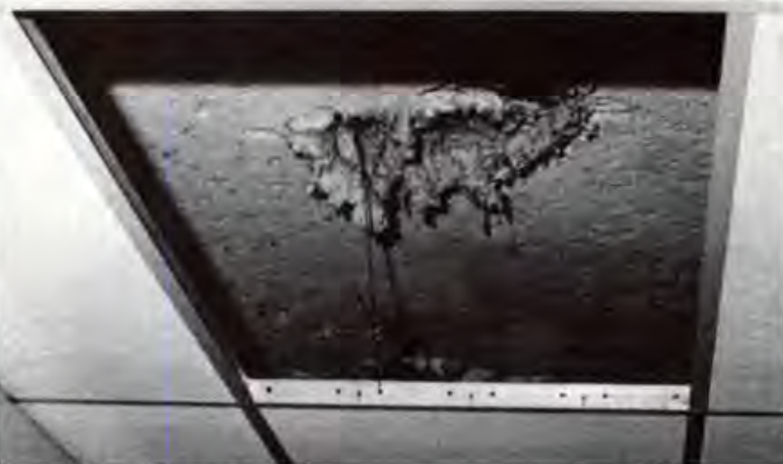
Friable asbestos above false ceiling.
