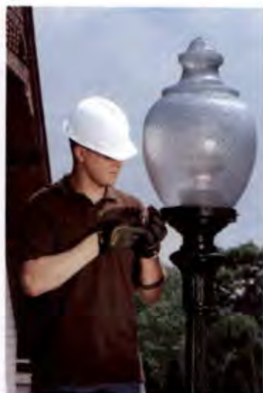
1. Loosen Set Screws
