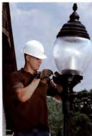
5. Connect Power to LED Conversion Kit
