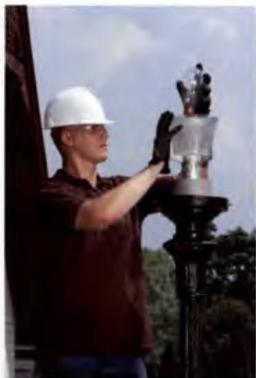
3. Remove Lamp and Refractor
