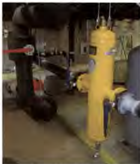
Spirovent Air / Dirt Separator Pummill Hall
