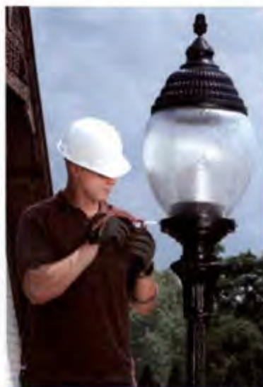
6. Tighten Set Screws
