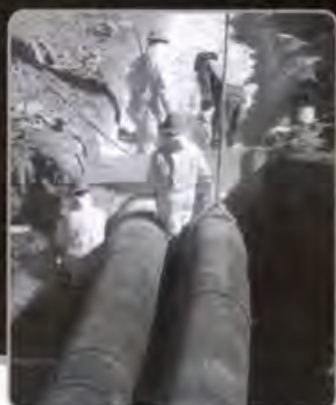
NATIONAL CENTER THERAPEUTICS MANUFACTURING - TEXAS A&M 24" HDPE CWSR INSULATED WITH GILSULATE®500XR A&M'S CAMPUS DISTRIBUTION MASTER PLAN FOR CWSR/HWSR RECENTLY CHANGED FROM PIF TO GILSULATE®500XR
