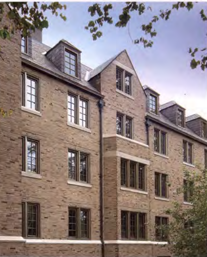
University of Notre Dame's historic Farley Hall renovation. The existing window frames were left in place and encapsulated with aluminum interior trim to preserve and restore the campus' architectural legacy.
