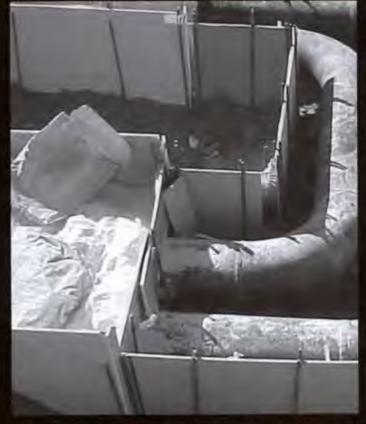
Gilsulate has insulated and protected underground pipes and tanks for over 60 years. This federally approved, patented system is economical, thermally efficient and hydrophobic. Gilsulate®500XR is load-bearing and provides a dry, stable environment for the long-term reliability of underground piping systems operating between 35° and 800° F. Examples of its many applications include steam, condensate, hot and chilled water.
