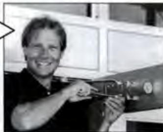
Install surface mount closer.
