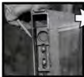
Replace old closer arm with pivot plate.
