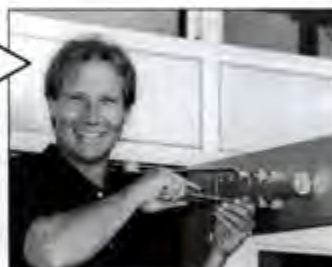
Install surface mount closer.
