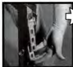
Replace old closer arm with pivot arm.
