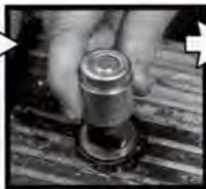
Slide cap over old closer spindle.
