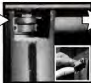
Rehang door and attach endload block.
