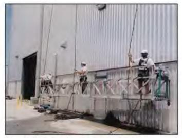
Figure 1. Inspection of wall using swing staging
