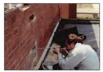
Figure 4. Performing a boroscope analysis to view wall cavity and related back-up wall
