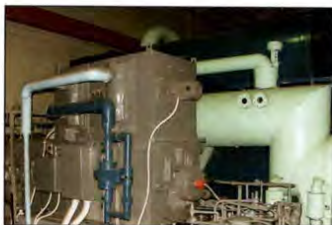
Main chiller plant: 1969 vintage 2000-ton machine slated for replacement
