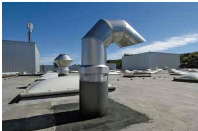
is an odor-free polyurethane (PUR) resin membrane system that is tinted throughout and color formulated to resist fading. Because there is no need to apply a separate topcoat over a membrane, the one-step application reduces labor and installation costs. To learn more, contact Kemper System at [www.kempersystem.net](http://www.kempersystem.net).
