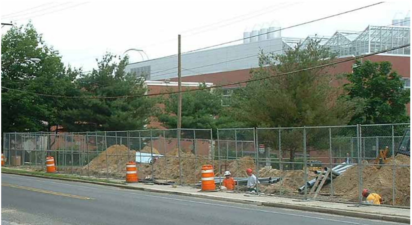
Utility infrastructure upgrades on a main campus roadway.
