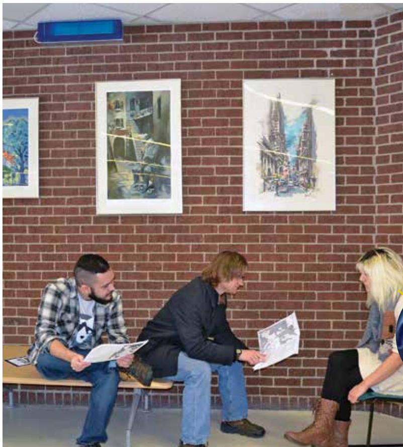
An upper-air UV light fixture (above) disinfects the air in the student lounge at Schenectady County Community College.
