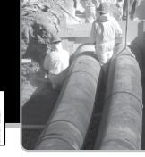
NATIONAL CENTER THERAPEUTICS MANUFACTURING - TEXAS A&M  $24~^{\prime\prime}$  HDPE CWSR INSULATED WITH GILSULATE 500XR. A&M' S CAMPUS DISTRIBUTION MASTER PLAN FOR CWSR/HWSR RECENTLY CHANGED FROM PIP TO GILSULATE 500XR.
