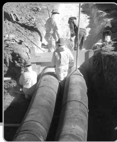
NATIONAL CENTER THERAPEUTICS MANUFACTURING - TEXAS A&M 24" HDPE CWSR INSULATED WITH GILSULATE®500XR. A&M'S CAMPUS DISTRIBUTION MASTER PLAN FOR CWSR/HWSR RECENTLY CHANGED FROM PIP TO GILSULATE®500XR.
