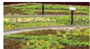
Extensive Vegetated Roofing System
