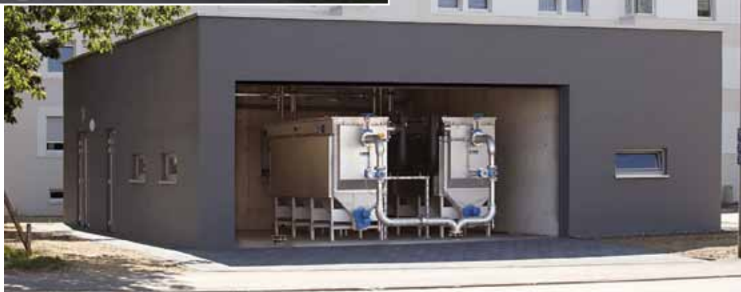
Apartment complex in Straubing, Germany using wastewater heat exchangers.
