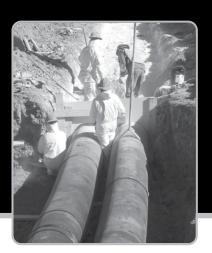
NATIONAL CENTER THERAPEUTICS MANUFACTURING - TEXAS A&M HDPE CWSR INSULATED WITH GILSULATE 500XR A&M'S CAMPUS DISTRIBUTION MASTER PLAN FOR CWSR/HWSR RECENTLY CHANGED FROM PIP TO GILSULATE\*500xr.
