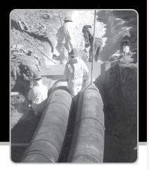
NATIONAL CENTER THERAPEUTICS MANUFACTURING - TEXAS A&M 24 " HDPE CWSR INSULATED WITH GLISULATE<sup>®</sup>500Xr. A&M' S CAMPUS DISTRIBUTION MASTER PLAN FOR CWSR/HWSR RECENTLY CHANGED FROM PIP TO GLISULATE<sup>®</sup>500X
