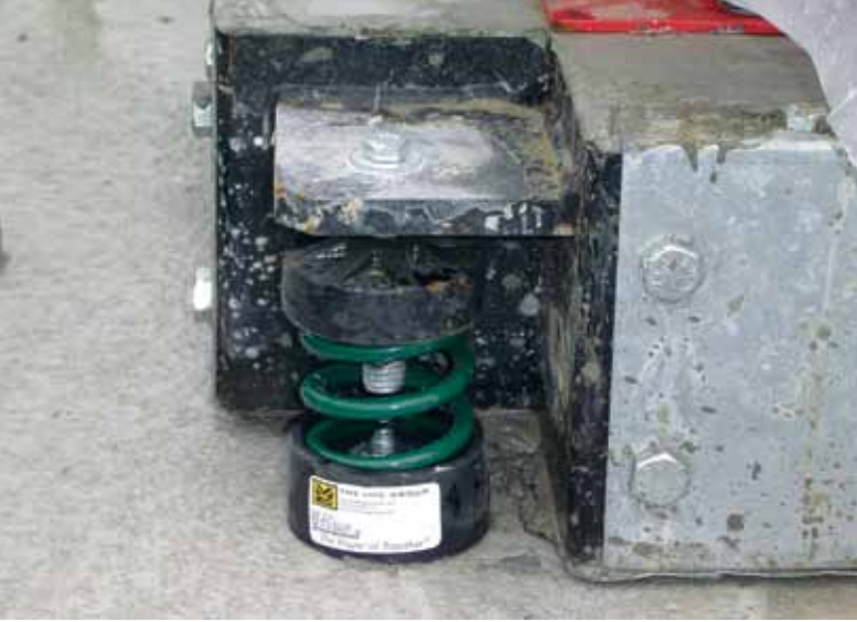
SPRING ISOLATOR SHORT CIRCUIT
