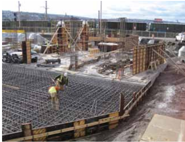
HEAVY FOUNDATION NEAR TRAIN TRACKS, UNIVERSITY OF SCRANTON
