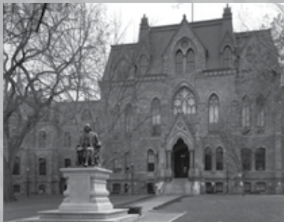
University of Pennsylvania Historic Stone Facade Repairs
