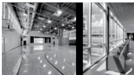
Manassas Park Elementary School | Manassas, VA Winner of Mid-Atlantic Construction's Best of 2009 K-12 Project of the Year LEED Gold Certification Pending
