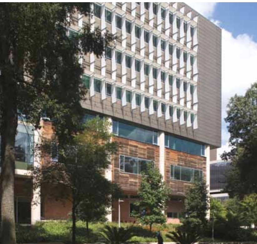
School of Nursing – looking southwest
