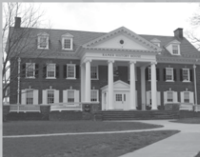
Lafayette College Interior Adaptive Reuse
