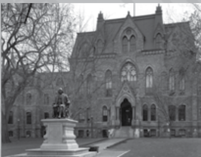
University of Pennsylvania Historic Stone Facade Repairs
