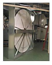
**Airxchange** announces its FA Series field-assembled cassettes dramatically reduce installation times and costs. Cassettes (wheels and frames) are factory-built, tested, marked for reassembly, and then disassembled for shipment. On-site assembly and installation are fast and easy, typically taking one day. Also,
