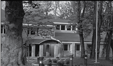
W.S. Cumby Office Complex • LEED Certified (2004)
