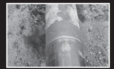
This is a tie-in on a steam line at a university. Note the old pipe was insulated and protected during it's original installation with **Gilsulate**<sup>®</sup> circa 1955-1960. The tie-in and new line will be insulated and protected with **Gilsulate**<sup>®</sup> **500XR**
