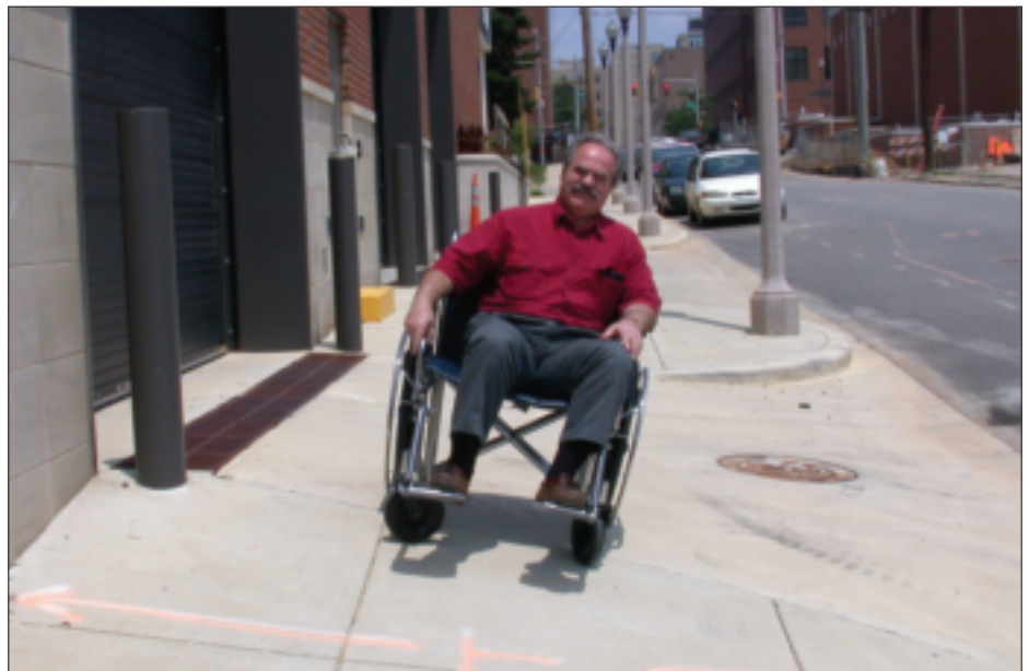
This cross slope is too steep and is an example of what happens when finish grades and spot elevations are not checked and confirmed by the design professional during construction.
