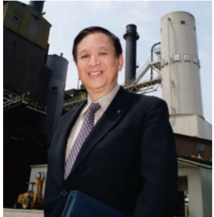
ISU's power plant has operated since 1906 and contains seven boilers, four turbine generators, and five centrifugal chillers.
