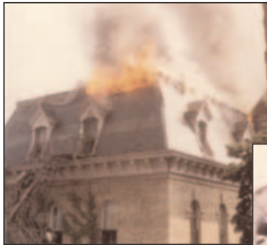
In 1979, Notre Dame University's St. Edwards Residence Hall caught fire while undergoing an extensive renovation.
