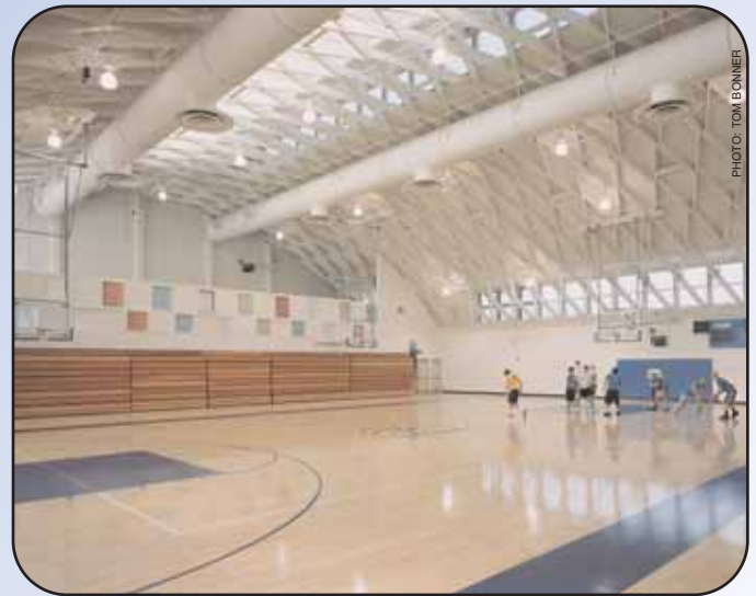
South Gymnasium with new clerestory glazing and ventilation system
