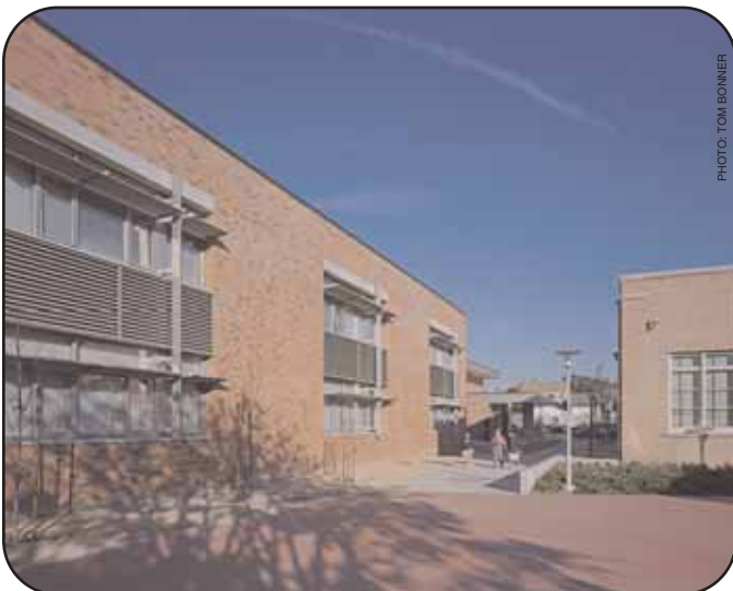
South side of Science Building
