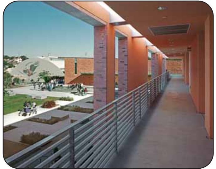
North side of Science Building looking toward Music Wing and South Gymnasium beyond
