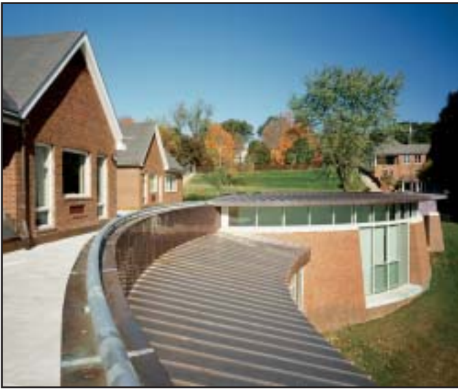
The new entry to the Fay School, Southborough, Massachusetts shown here reoriented the flow of circulation in the building. The new brick matched the original brick but the curvilinear geometry was used to soften the sawtooth geometry of the roofs.
