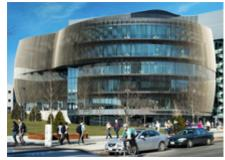
Northeastem University's new 234,000-square-foot Interdisciplinary Science and Engineering Complex (ISEC), designed by Payette and implemented by Arup, used an integrated design process, advanced energy modeling software, and building information modeling (BIM) to create a high-performance, energy-efficient laboratory facility.
