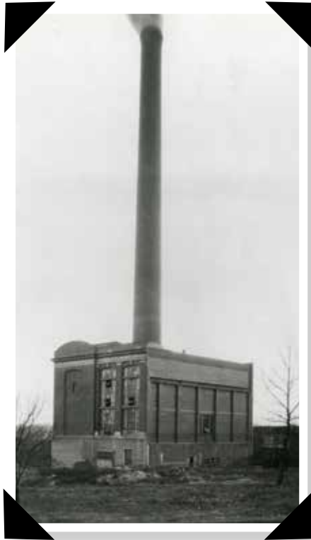
Ohio State College (now University) power plant, 1917. The plant was expanded several times and renamed McCracken Power Plant for APPA's 1924 president William C. McCracken.
